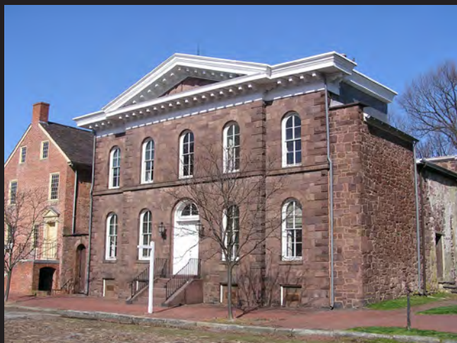
Fig. 25. Sheriff's House, New Castle, now part of the First State National Historic Park
